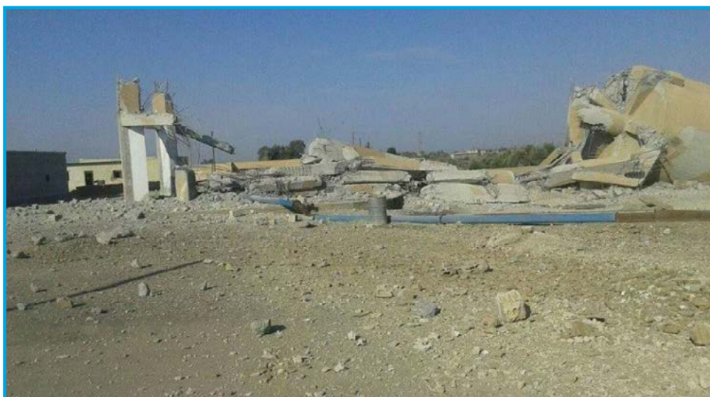
The destruction in the water tank in the aftermath of a bombing by fixed-wing international coalition forces warplanes in al Ghassaniya village, al Raqqa – March 8, 2017
