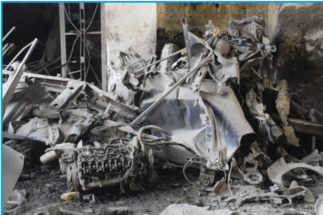
Damages in the aftermath of a shelling by Syrian regime forces on a car garage belonging to the local council in Douma city, Damascus suburbs – January 13, 2018
