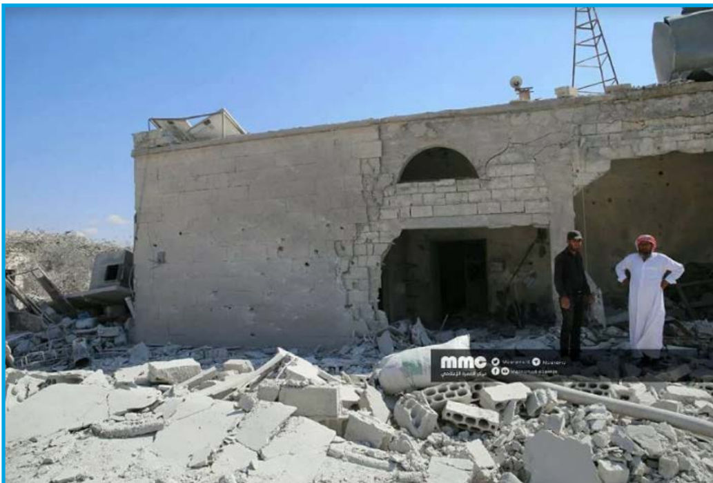
Destruction at al Janoubi Mosque in the aftermath of a Syrian regime bombing in Mazra'at al Tes'a, Idlib – September 28, 2017
