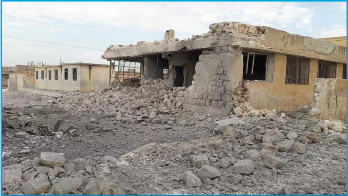
Destruction in the aftermath of a barrel bomb attack on a school area in Babolin village – December 28, 2017
