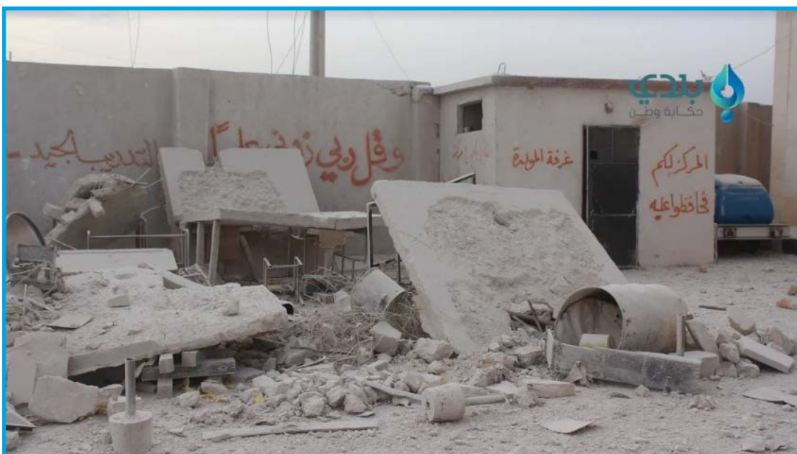
Destruction at the civil defense's preparation and training center in the aftermath of an attack by warplanes we believe are Russian in al Aatareb city – November 13, 2016
