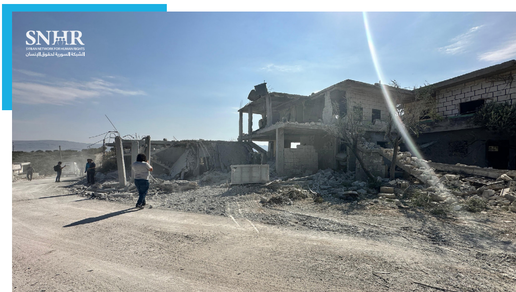
👁 Destruction caused to houses in Jafatlek Haj Hammoud village in Idlib by a Russian aerial attack - October 6, 2023 © SNHR
